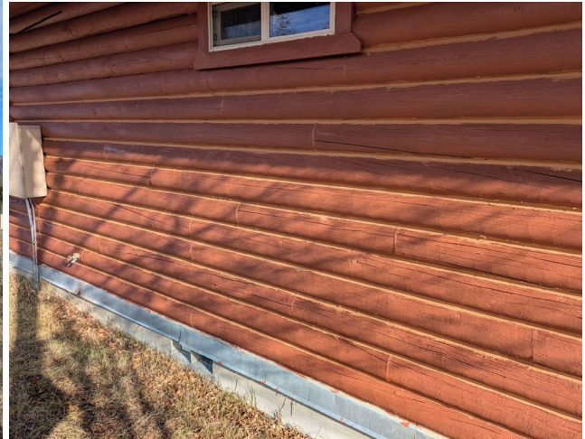
Finished staining all Module cabins and started log jamming.
